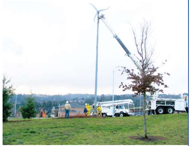
Salem Electric line crew assisting with the assembly and installation of the wind generator.
