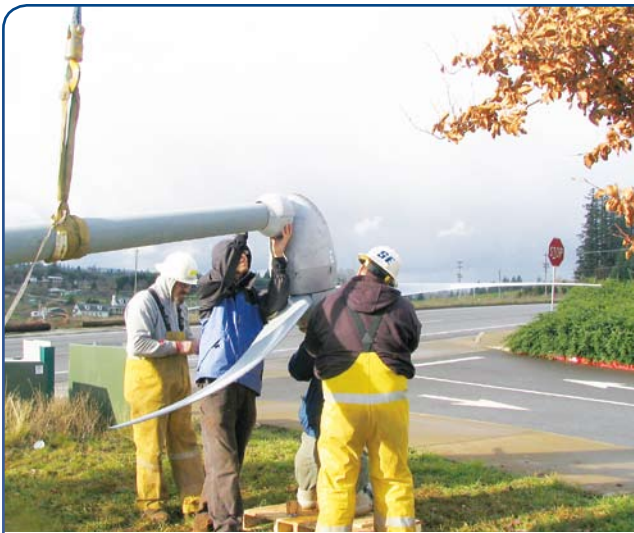
Salem Electric line crew assisting with the assembly and installation of the wind generator.
